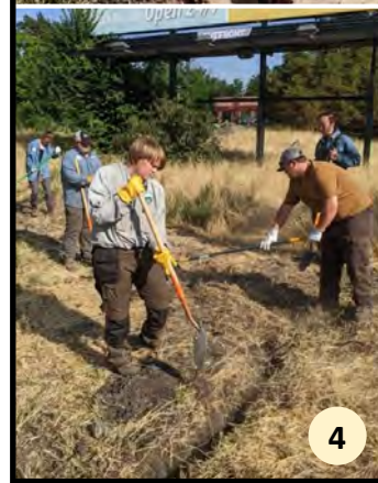
Images: 1.) Mark Casebier using the trenching machine for 1500 feet!!! 2.) It took A LOT of volunteers A LOT of time to cover the pipe for 1500' in ditches. 3.) Greg Christensen , amazing volunteer, readying the ditch to carry the 2" polypipe. 4.) Integral Youth Services (IYS) crew covering the polypipe that will bring water to 128 plants along Ken Hay trail and Highway 97. 5.) An oak tree planted in Memory of Ben Kerns near the junction of the Ken Hay Trail and the railroad bed.
