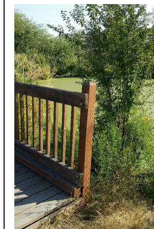
Post 12-Bridge, No. end
