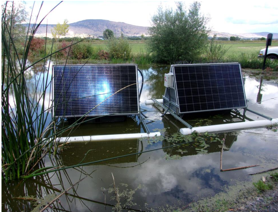
Solar-powered pump project funded by the Schwemm Family Foundation THANK YOU!
